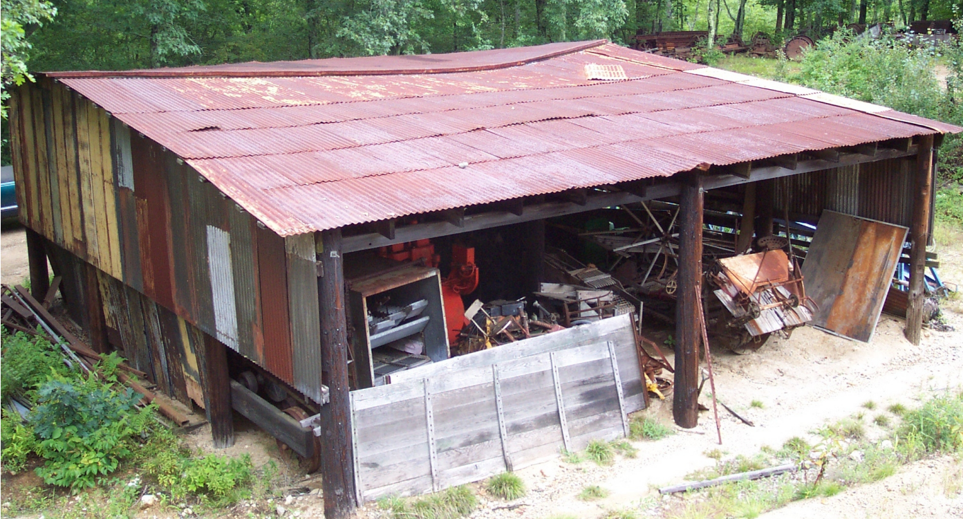
Drying Shed – View from Back Side Prior to Restoration (Aug. 2011)
