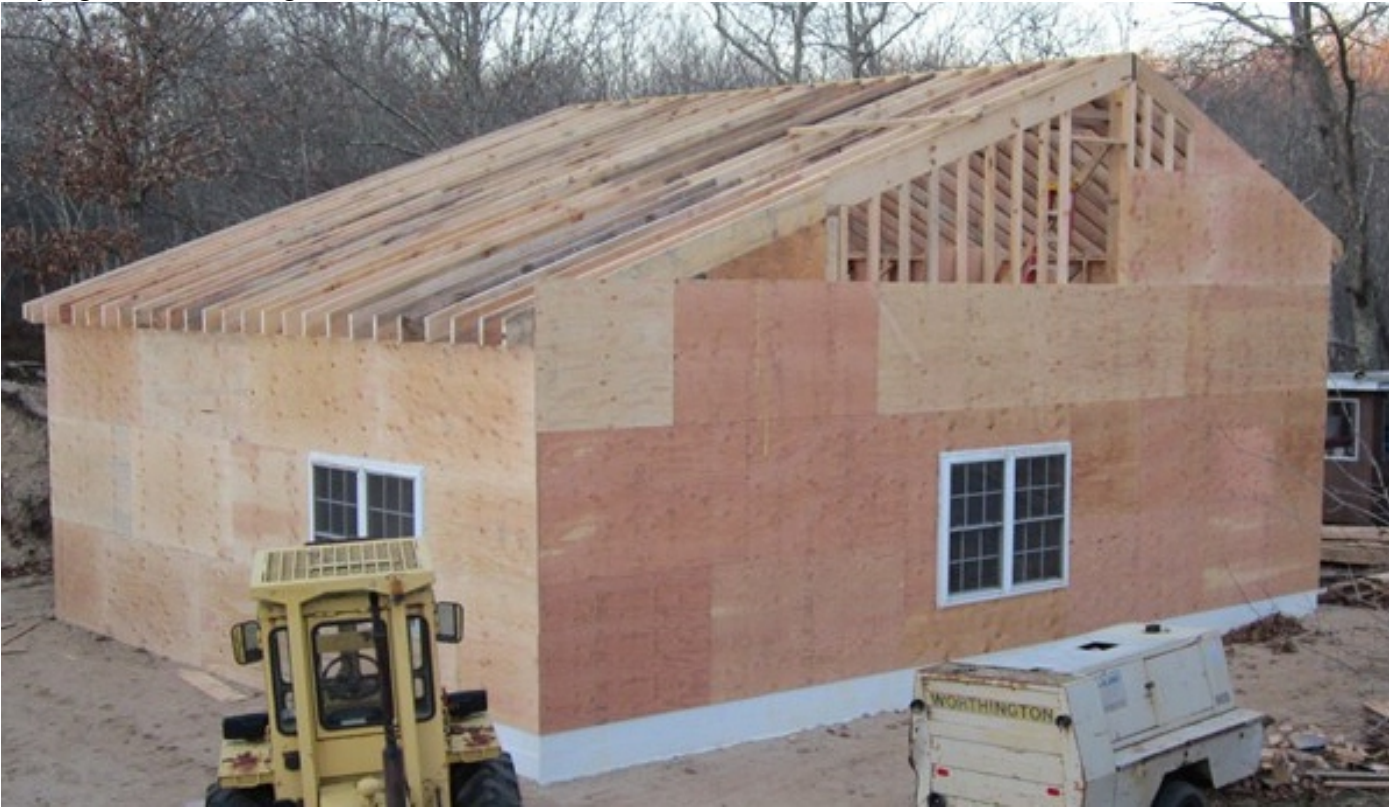
Drying Shed Nearing Completion Nov. 2012
