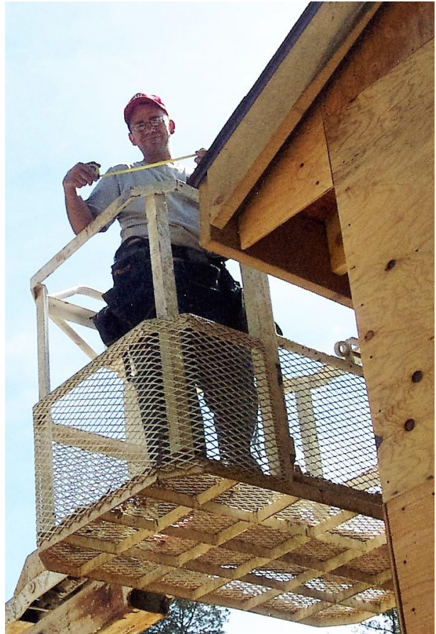
Dave Chester utilizing the apple picker which came in very handy as a manlift
